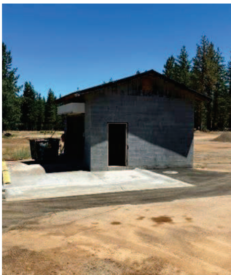
Headworks Apron Extension
