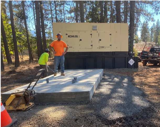
Preparing the pad for the new Generator
