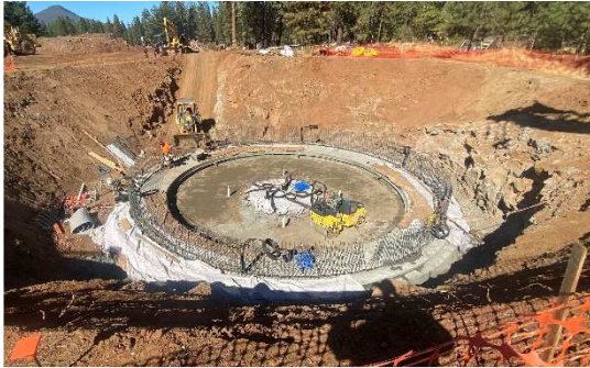
Construction of the new Clarifier
