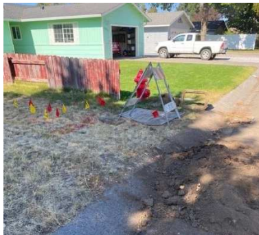
WhiteHawk Construction installing new radio read meters
