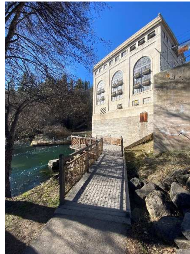
Hat Creek Powerhouse No. 2 built in 1921 and was commissioned Sept. 28, 1921
