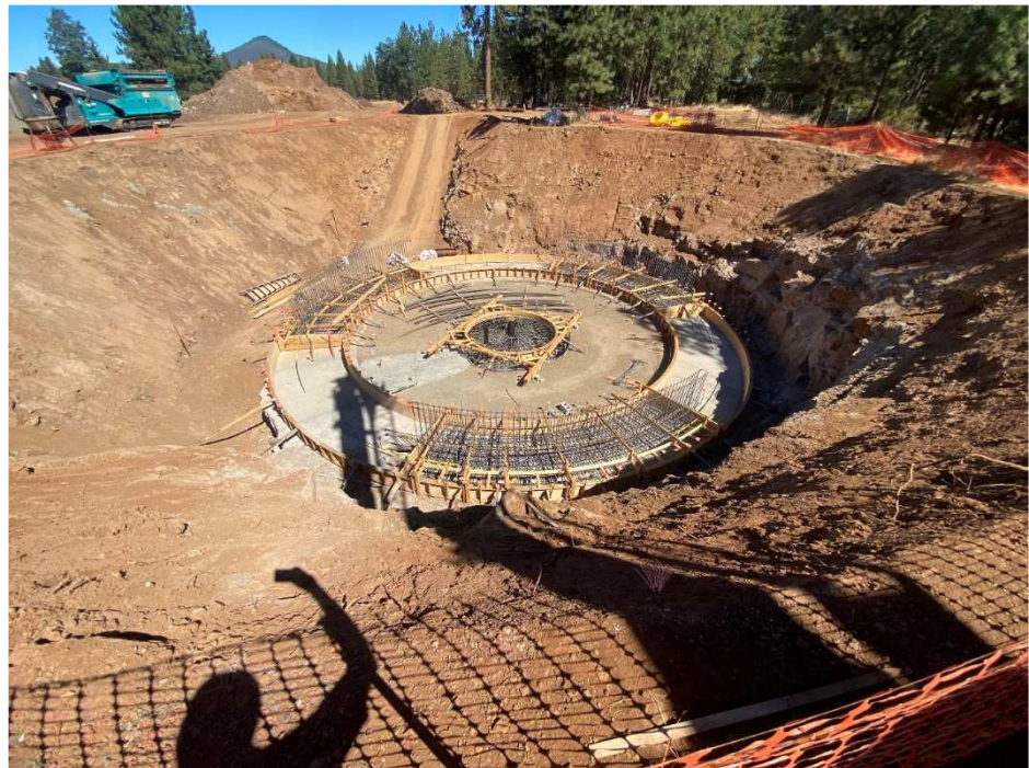
Clarifier rebar and formwork
