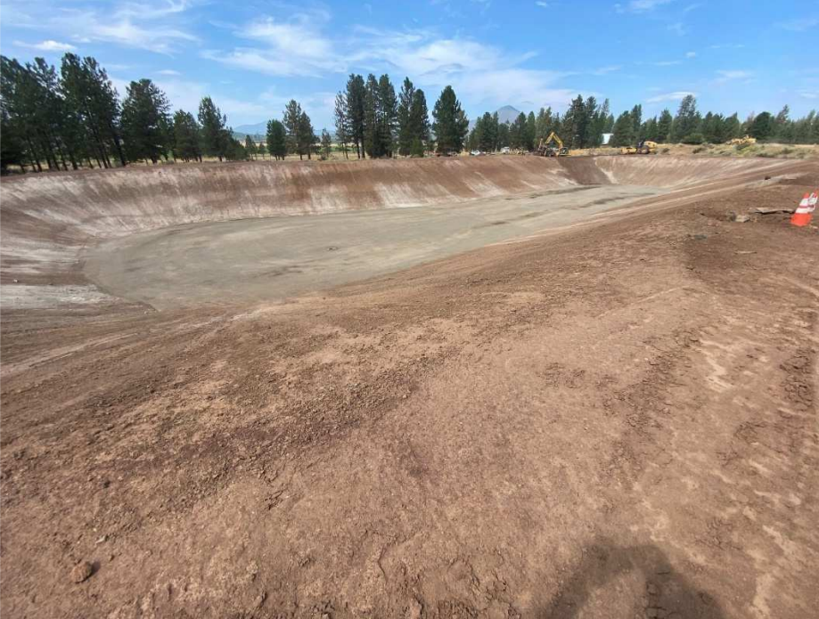
Sludge Lagoon Grading
