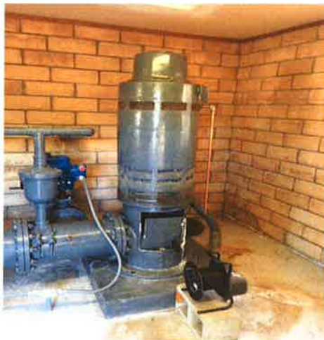
Well #6 Pump-house and Vertical Turbine Pump
