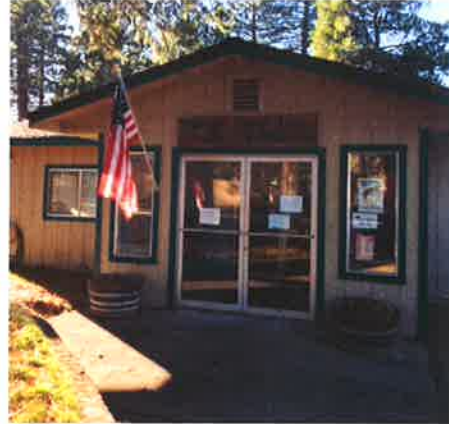
Burney Water District Office
